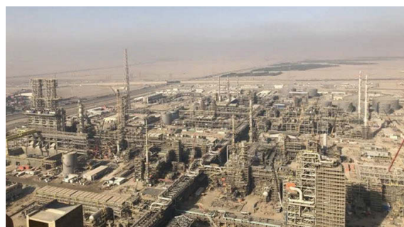
(Photograph courtesy of JGC Corporation)
